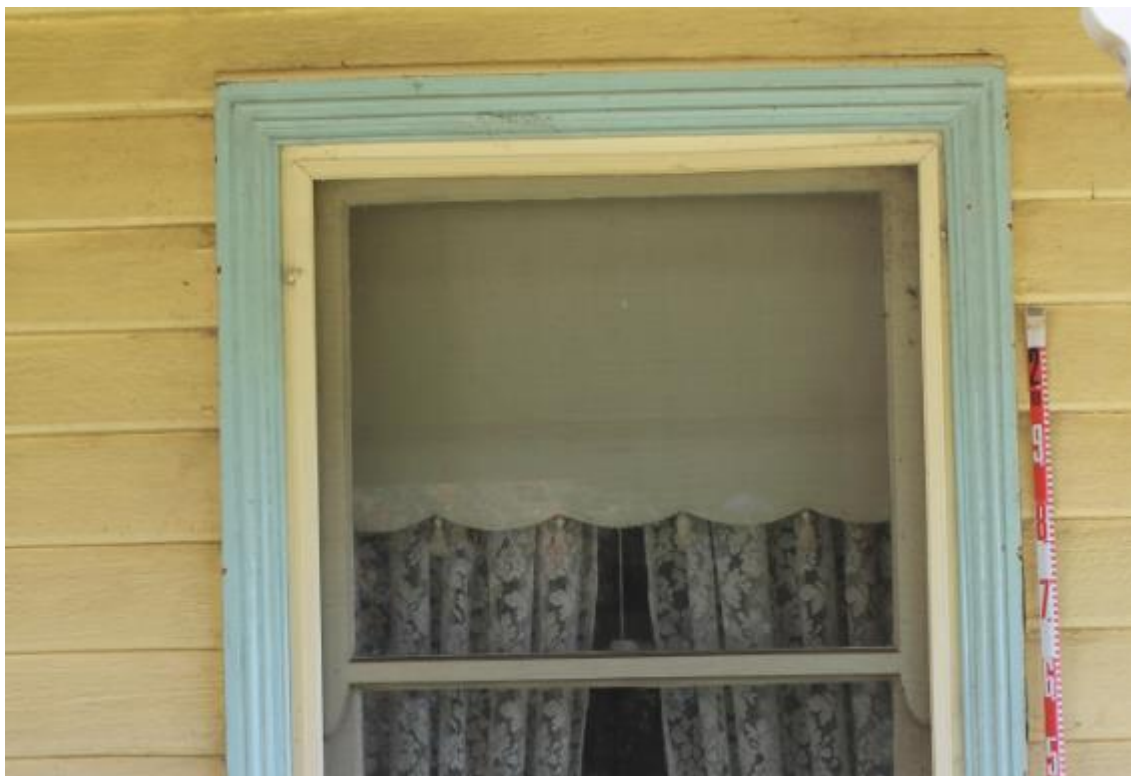
Plate 8 Cladding and window on southern façade (source: AECOM 2020)
