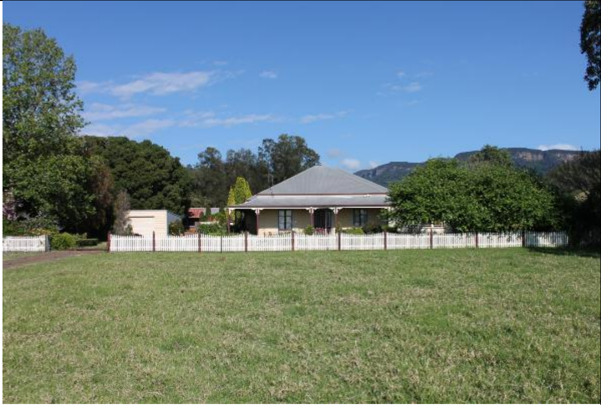
Plate 5 View east showing front facade of homestead and entry (source: AECOM 2020)
