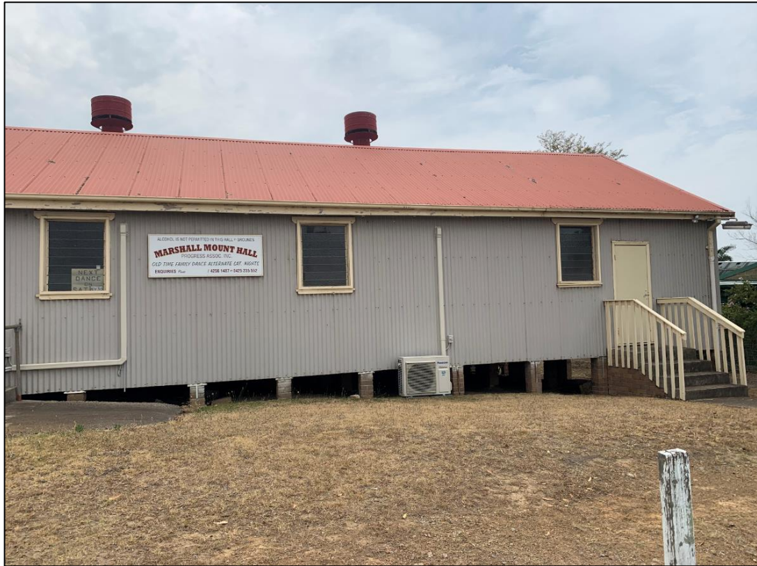
Plate 1 View north showing Marshall Mount Hall (Source: AECOM 2018)
