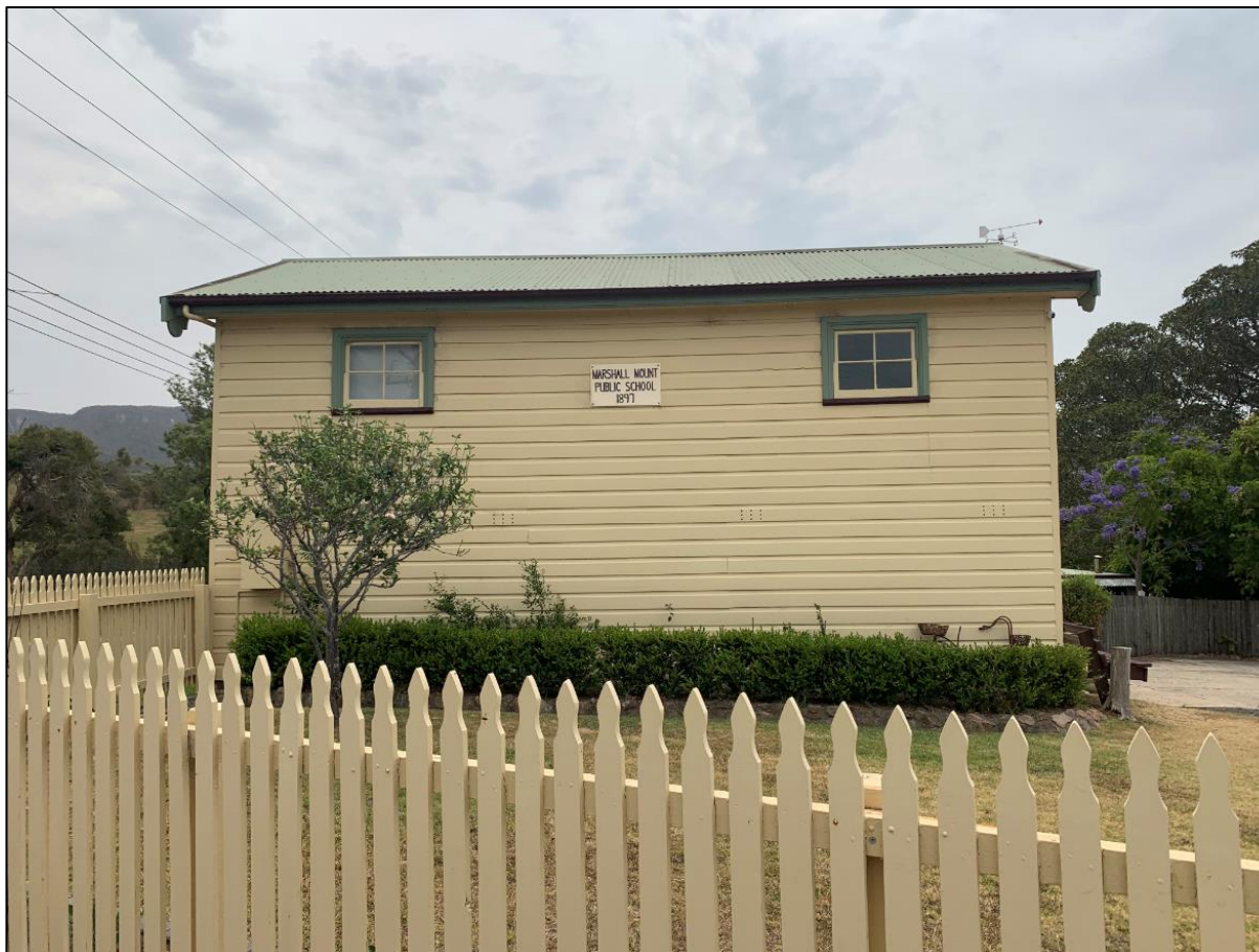
Plate 4 View north of Marshall Mount Public School (Source: AECOM 2018)
