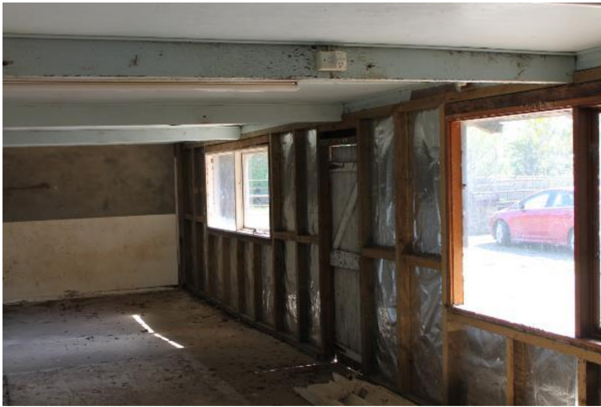
Plate 12 Internal dairy showing timber framework on front façade (source: AECOM 2020)
