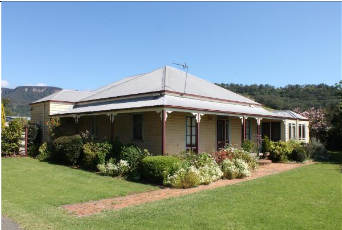
Plate 6 View northwest showing front and southern side of homestead (source: AECOM 2020)
